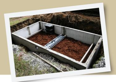
A septic system is an individual wastewater treatment system using soil to treat small wastewater flows from a home or small group of homes. There are two parts to a conventional system:
